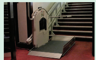
Leisure centre installation
