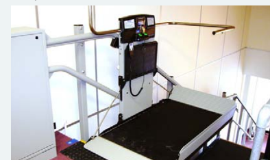
Council building installation in Wales
